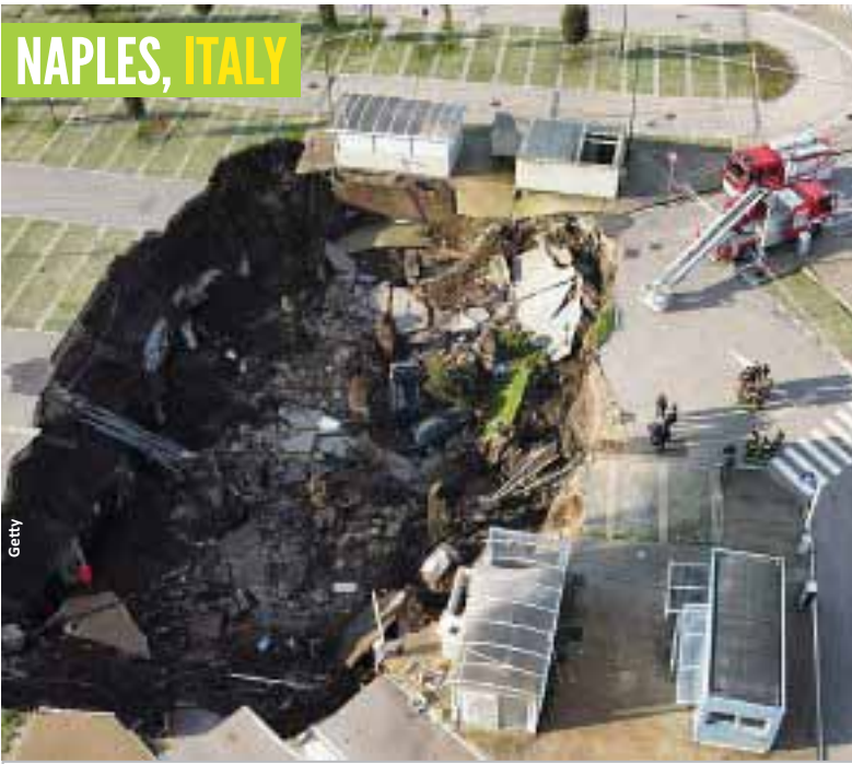
THIS huge sinkhole opened up in a hospital car park, after the ground beneath the park gave way.
